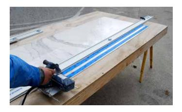
Cut back panels to total width of back wall minus 3/8". For instructions on how to cut Curava panels see section on "CUTTING CURAVA PANELS".
