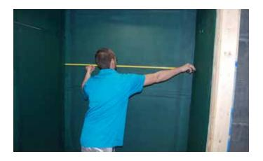
Measure width of back wall first. Deduct approx. 3/8" from the width of the back wall where it is narrowest. This will be the final total dimension of the back panels. For example if the back wall measures 59.5" at the narrowest point the back panels should add up to 59.125" (59.5" minus 0.375"). This space allows for the possibility of the back wall being out of square. The side panels will cover whatever gap is left between the back panels and the left and right side walls.
