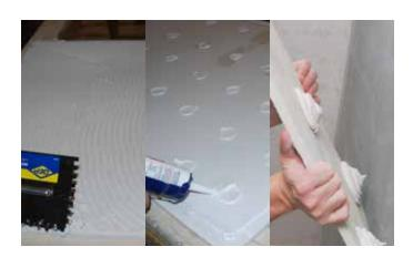
Ensure that all surfaces are clean, dry and free of dust before applying adhesive. Apply adhesive to the back of the panel as outlined in section "CHOOSING AN ADHESIVE".
