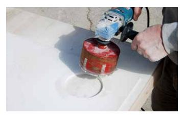
Measure exact location and size of cut-outs required for plumbing. Use diamond core bits or blades to make cutouts.
