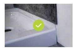
The bottom of the backer board substrate (cement board) should rest on top of the lip of the shower pan or tub deck lip
