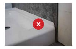
In no case should the cement board be installed behind the lip of the shower pan or tub deck as this can result in water leaks
