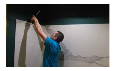
If there is a small gap, it can be filled with silicone and you have the option of using inside corner trim as well.
