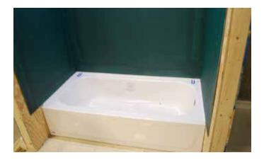
Place horseshoe shims at back corners of tub or shower base so that the back panel will rest on the shims and not directly on the tub or shower base.
