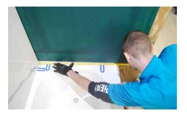
Measure required width and height of side panels. Width should be measured from back wall to edge of tub or shower base. Remember that you have the option of using 1.5" wide trim if needed.
