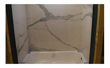
Now that the panels have been installed caulk around perimeter of panels, including at inside corners and between tub or shower base and bottom of panels.
