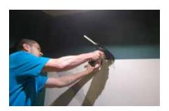
Once back panel is straight, plumb, and level, use a hot glue gun to keep the panel in place while adhesive cures.
